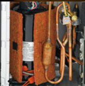
Sound-proof Material The compressor is thoroughly protected to prevent annoying noises.
